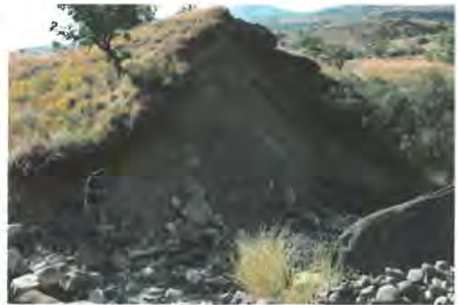
Figure 5: Erosion of the toe near the left flank exposes angular boulders within the soil which indicate a colluvial deposit.
