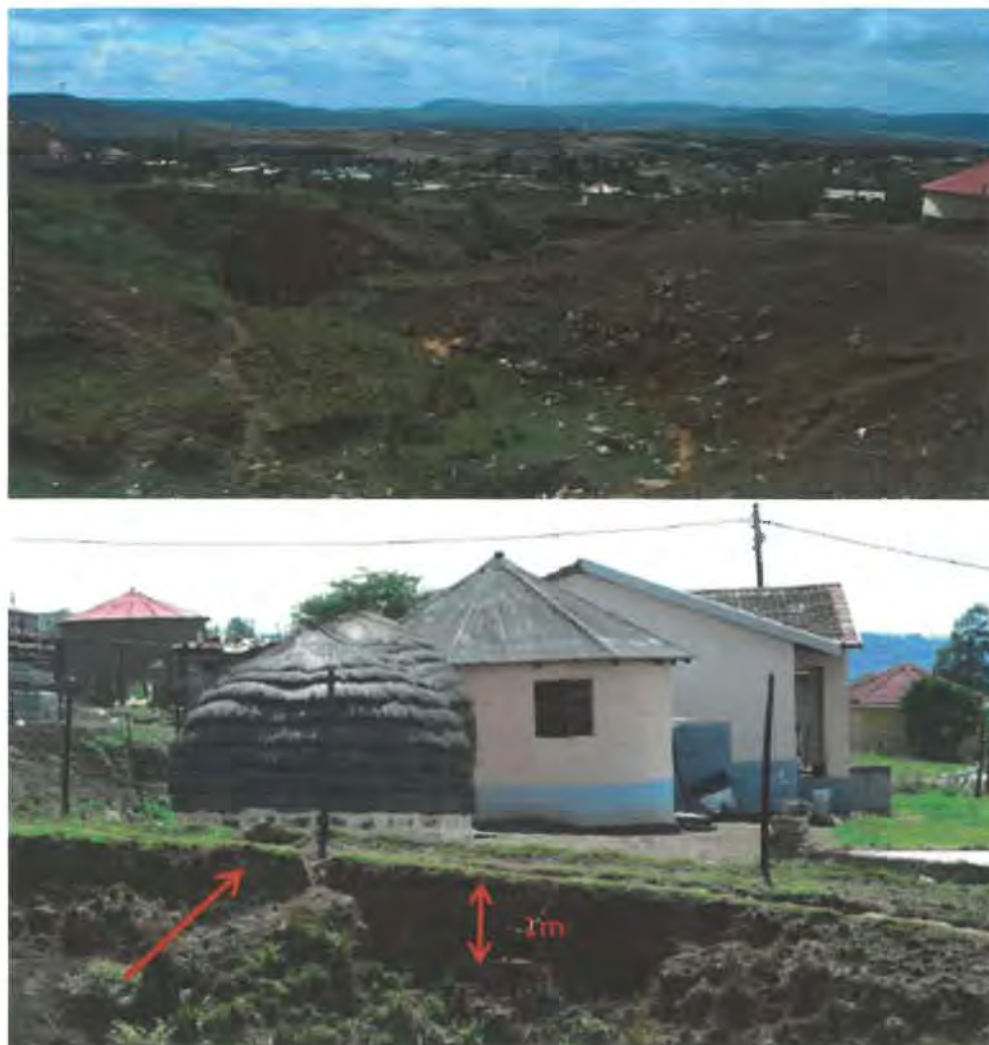
Figure 6 The sidewalls of the main gully retreat, to the extent that they then threaten the stability of dwellings and infrastructure (upper and lower image). Note that the 'step' some 1,5 m away from the boundary fence is already up to 1m high in places (lower image).
