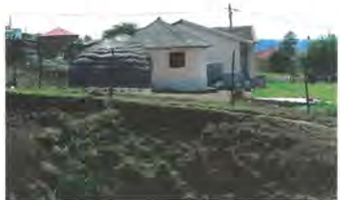
Figure 4: The steep gully sidewall is rapidly encroaching on a dwelling in the greater Ulundi area, threatening the safety of the inhabitants.
